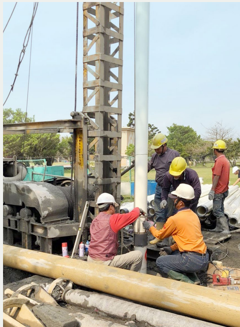
鑿井工程 Well drilling engineering
