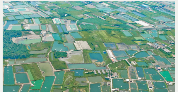
養殖輸水工程 Water Supply engineering
